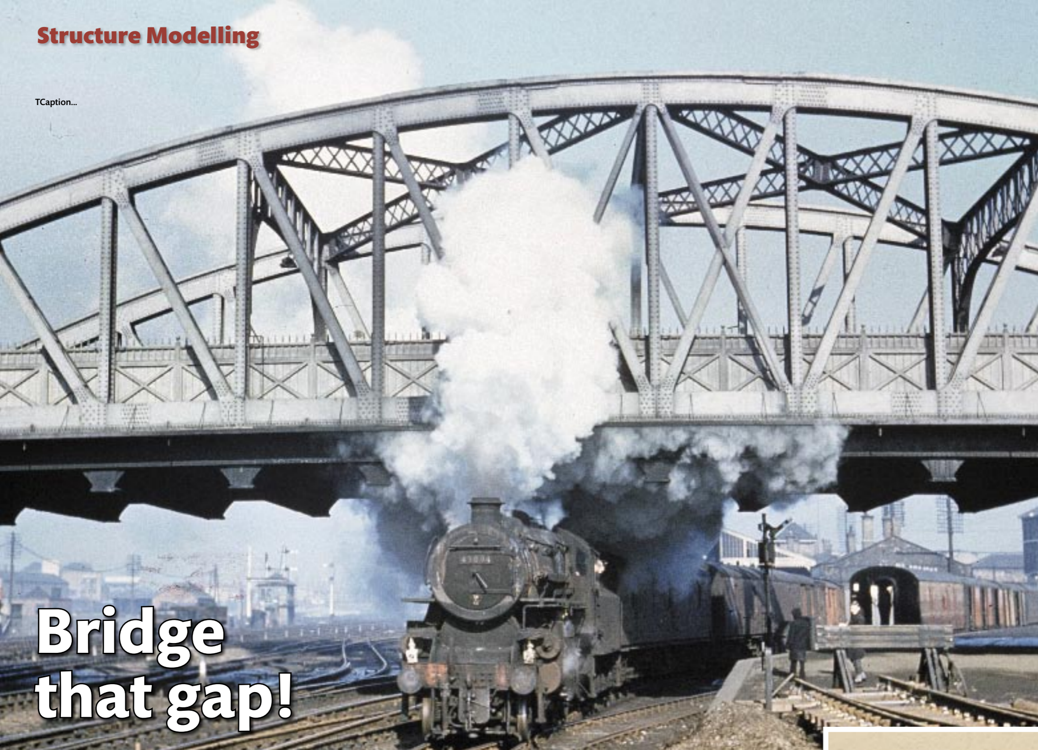
The classic American Warren truss was patented in 1848 by its designers James Warren and Willoughby Theobald Monzani. Its configuration combines strength with economy of materials so it can therefore be relatively light. Barry Cole
