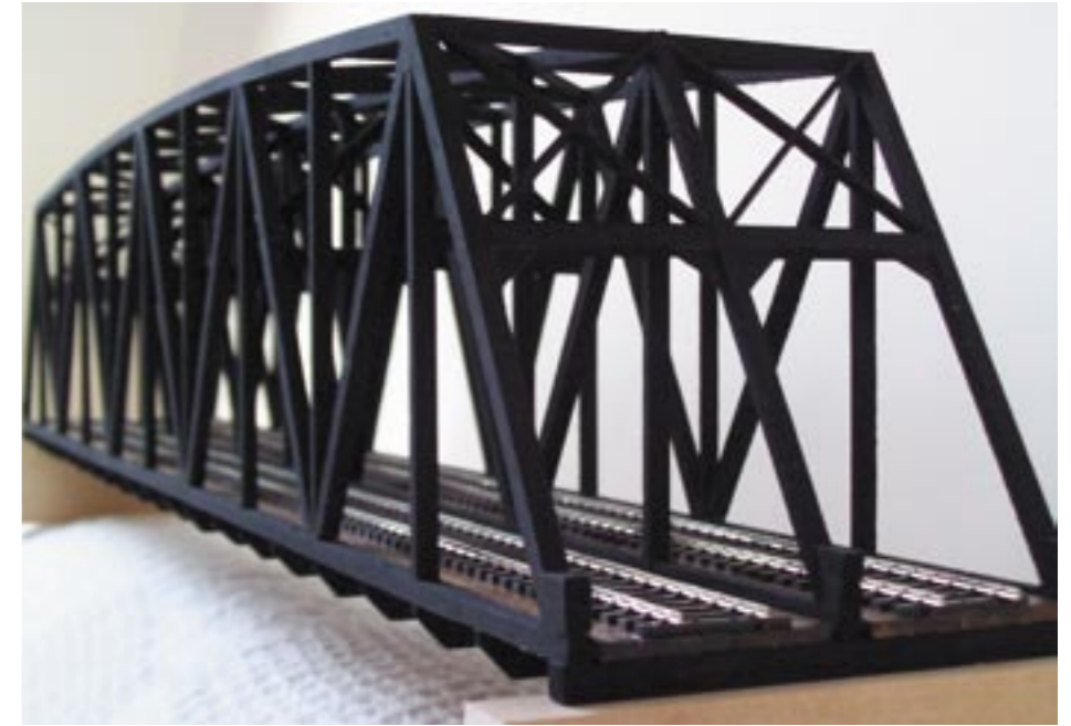
The classic American Warren truss was patented in 1848 by its designers James Warren and Willoughby Theobald Monzani. Its configuration combines strength with economy of materials so it can therefore be relatively light. Barry Cole
